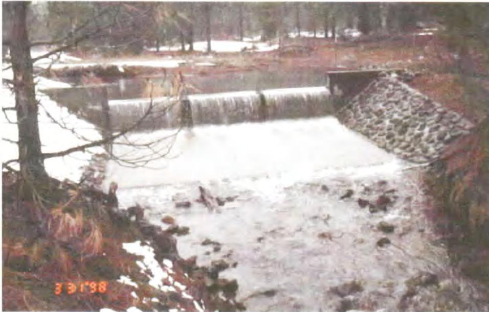
**Figure 9.** Spawning barrier constructed in 1997 near Christie Campground on Little Merrill Creek.
